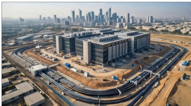
A modern, state-of-the-art data center facility under construction near a city. (Photo: Kabelo Mokoena)
